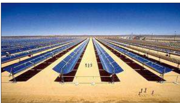
Fig 1: Trough solar thermal power generation system
